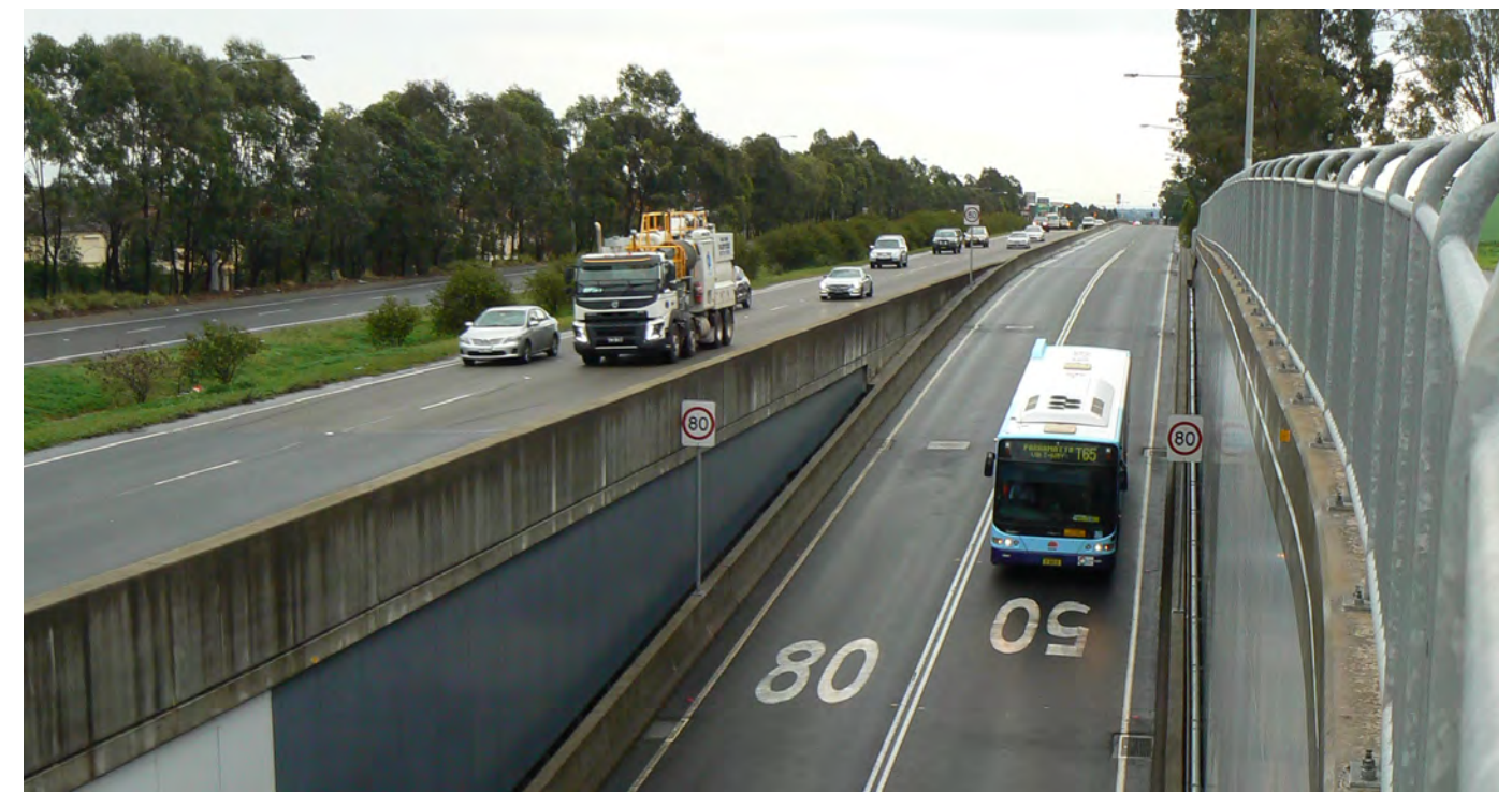
T-Way underpass, Windsor Road, Bella Vista
